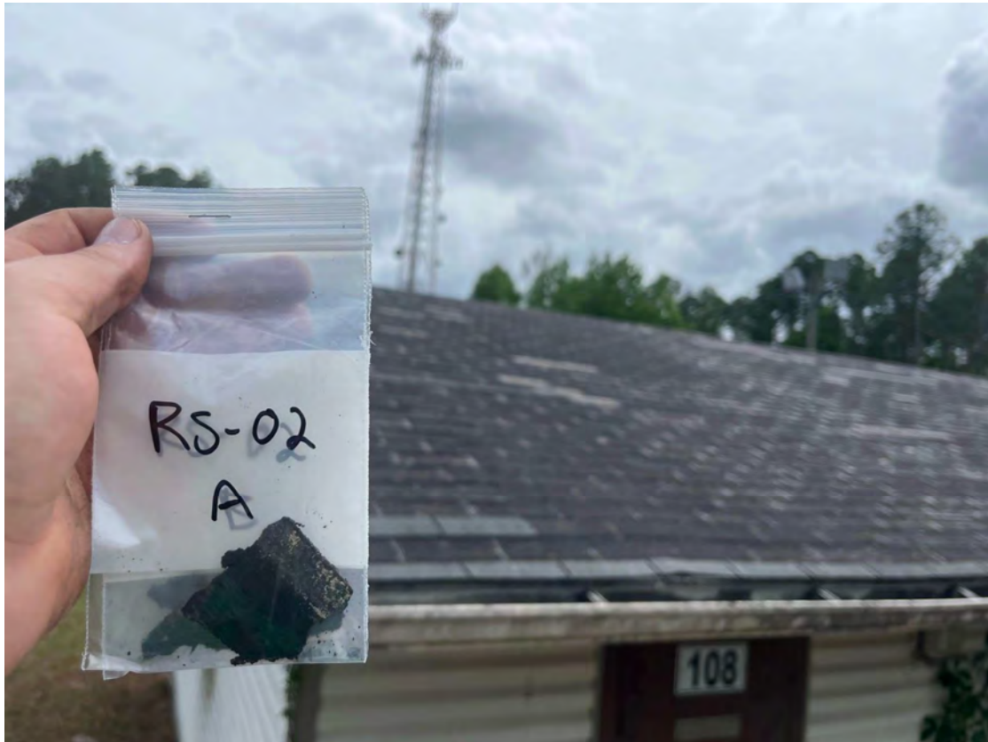
Upper Photo: RR-03-Black Rolled Roofing (Roofs)
