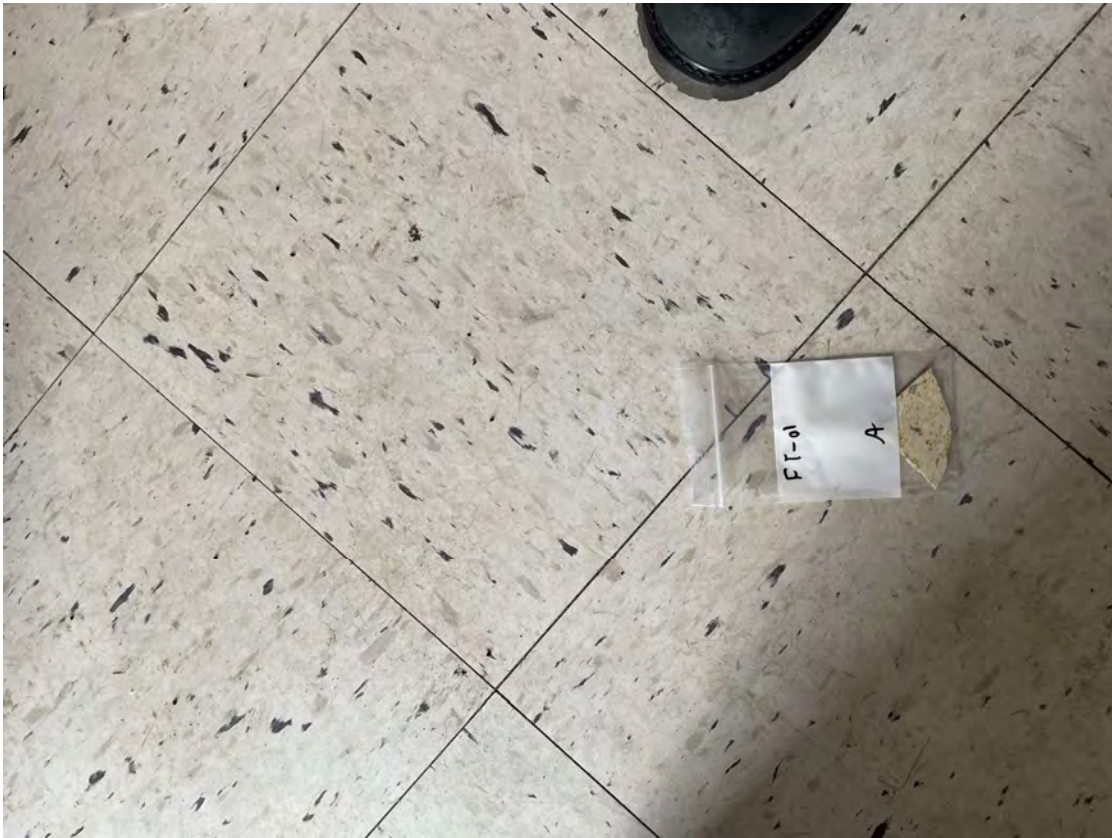
Upper Photo: FT-01-12" x 12" White Floor Tile with Black Mastic (Bldg. 10)
