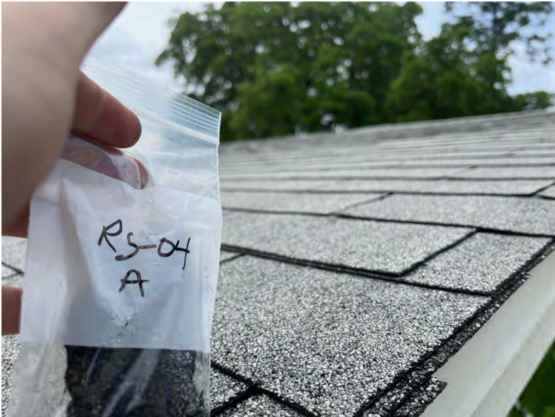
Upper Photo: RS-03-Black Roof Shingles (Roofs)
