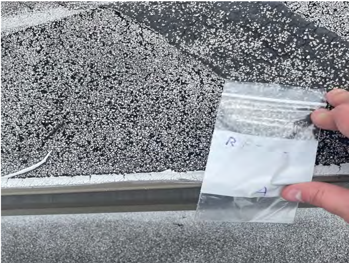
Upper Photo: RF-01-Black Roof Flashing (Roofs)
