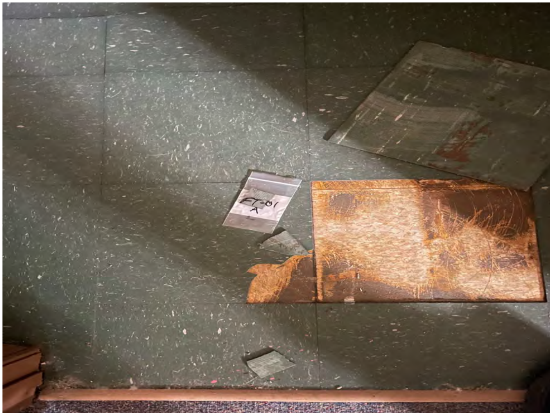
Upper Photo: DW-01-Drywall and Joint Compound (Bldg. 4)
