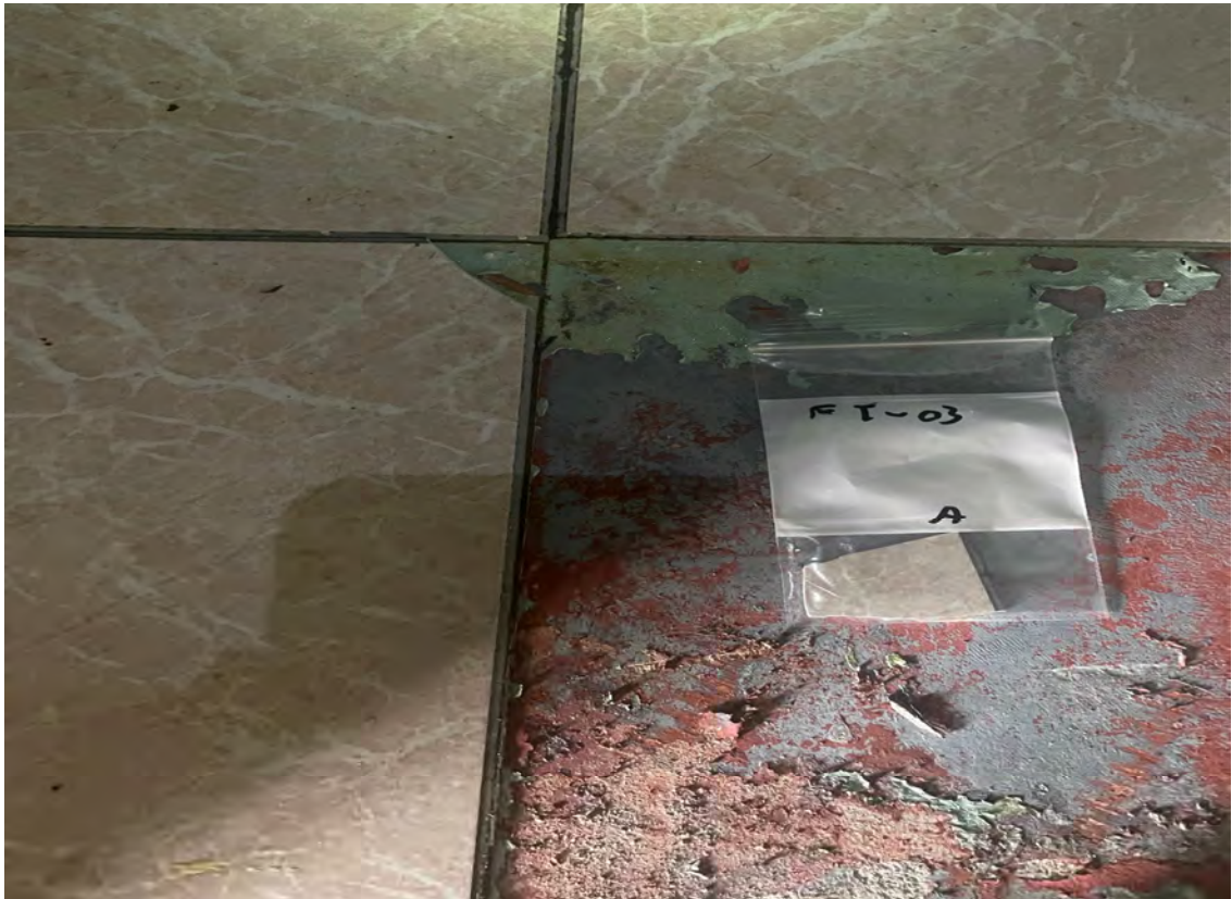
Upper Photo: FT-02-Gray Grout associated with Gray Ceramic Floor Tile (Bldg. 1)
