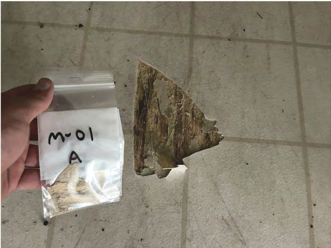
Upper Photo: FT-01-12" x 12" Beige Floor Tile with Tan Mastic (Bldg. 6)
