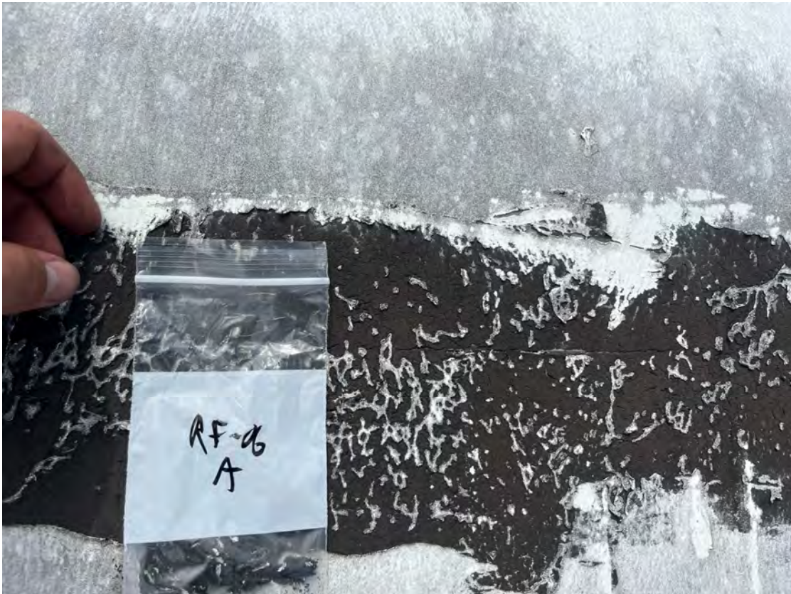
Upper Photo: RF-05-Black Roof Flashing (Roofs)
