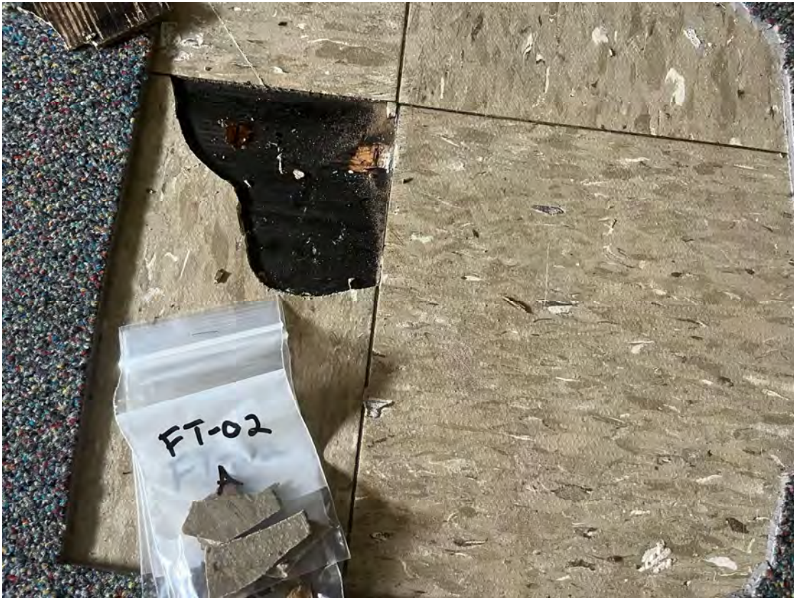
Upper Photo: FT-01-12" x 12" Green Floor Tile with Clear Mastic (Bldg. 3)
