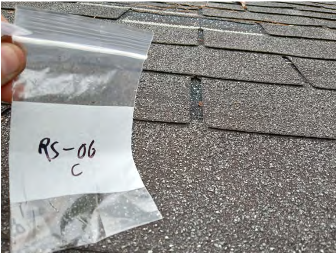
Upper Photo: RS-05-Black Roof Shingles (Roofs)
