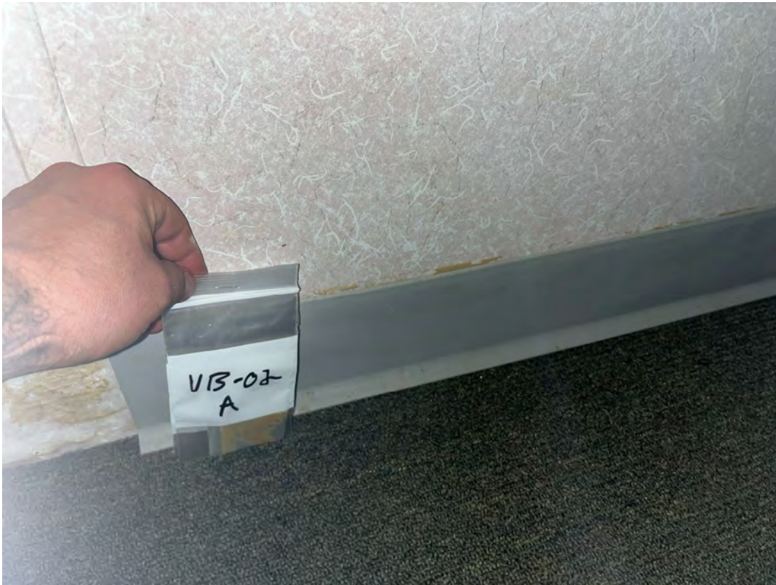
Upper Photo: VB-01-4" Tan Vinyl Cover Base with Tan Mastic (Bldg. 9)
